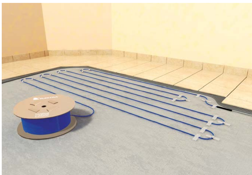
Initial fixing of the heating cable utilising self-adhesive tape
