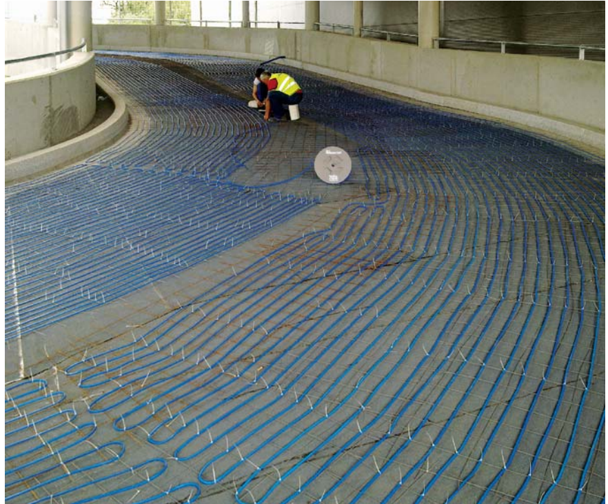
Fixing heating cable to installation mesh
