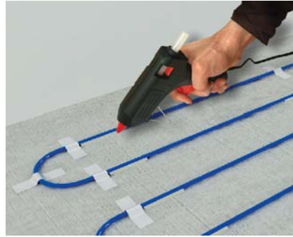
Fixing of the heating cable utilising of hot glue
