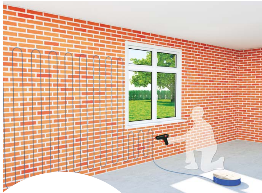
Fixing the ELEKTRA heating cable with hot glue
