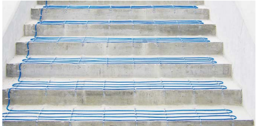
Example of ELEKTRA heating cable layout
